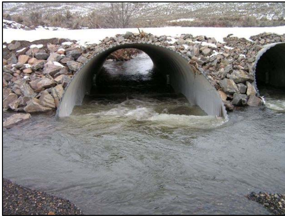
Irrigation diversion on Maggie Creek Ranch designed to allow for fish passage and provide for irrigation needs of the ranch. Photo credit – Bureau of Land Management
